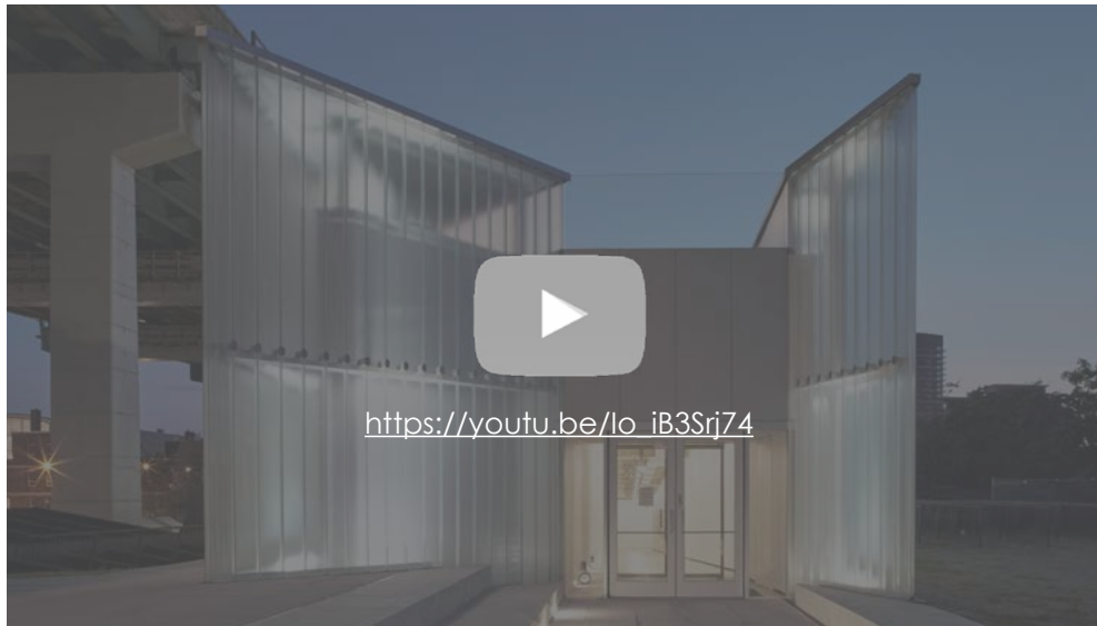
Fort York Visitor Centre, Toronto, Ontario, Canada by Kearns Mancini Architects & Patkau Architects. A “ghostly,” translucent, expansive channel glass rainscreen defines the building and offers a robust layer of protection against wind and moisture.
