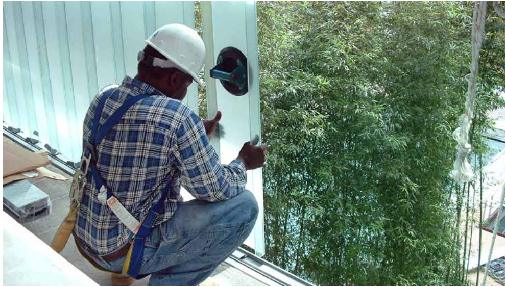
Espirito Santo Plaza Parking Structure, Miami, FL by Kohn Pedersen Fox Associates.
