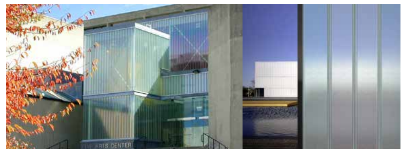
Low-E Thermal Performance Coating Iridescent Aesthetic, U-Value of 0.41
